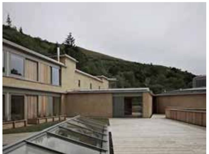
Figure 4: View Over Courtyard Towards Study Rooms.
