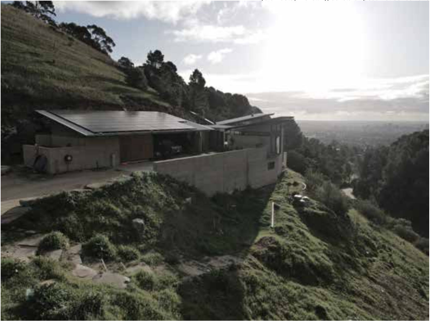
Adelaide Rammed Earth House: Kurna/Mount Osmond
