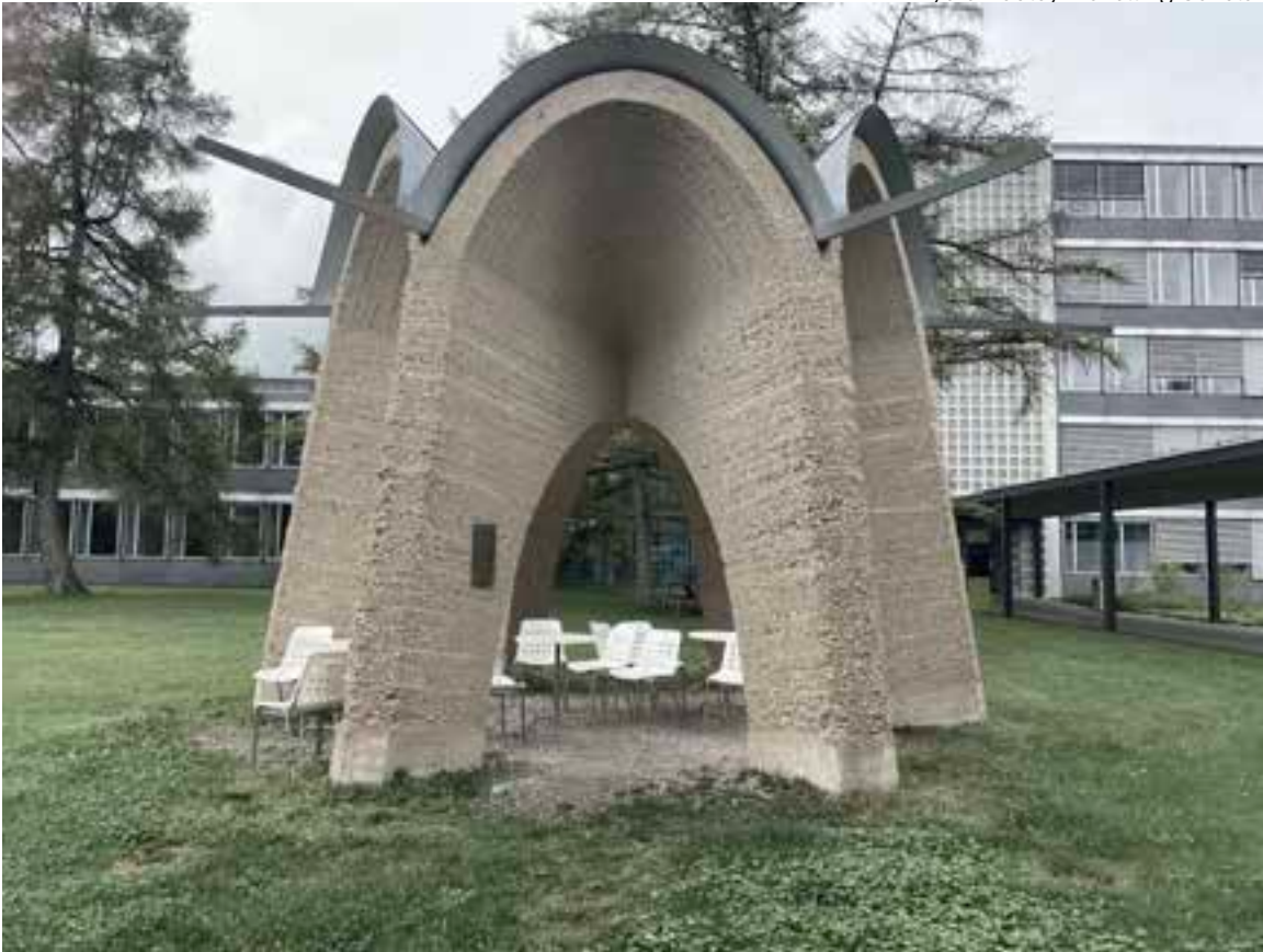
Rammed Earth Dome: Honggerberg, Zurich
