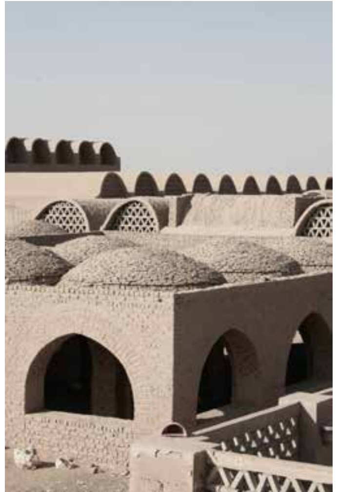
Figure 26: Fathy's New Baris public buildings, 1967, with a museum in foreground and market vaults to rear. The Mashrabiya windows are made from earth.
